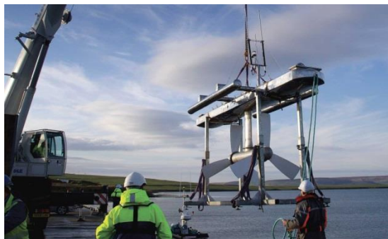
Figure 2. Magallanes Project turbine installation
